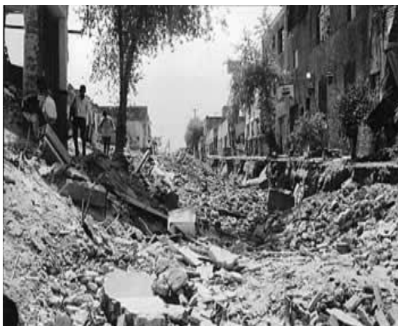
Rubble in center of street destroyed by sewer explosions in Guadalajara, 1992. Photo credit, with permission (Jon Seals): Disaster Recovery Journal at: http://www.drj.com/drworld/content/w2_028.htm ; accessed May 5, 2006.
